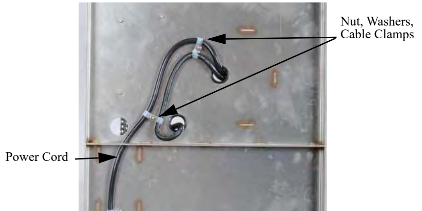
Underside Of Frame
