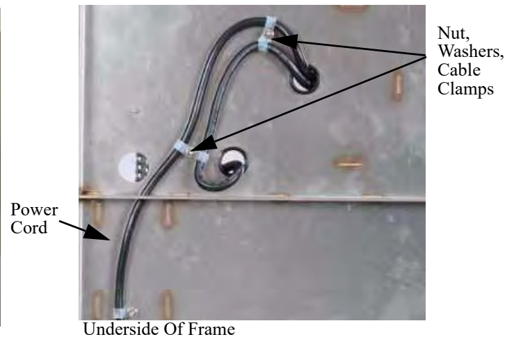
Underside Of Frame
